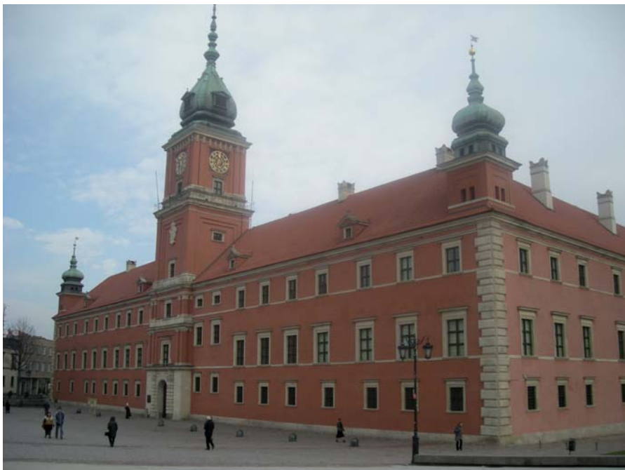
The Royal Castle in Warsaw has KATKO switches installed in it.
